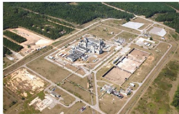
SRS P-Reactor Area Closure Project
