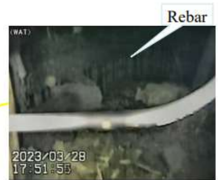
Photo 1: Point ⑧ at pedestal base
