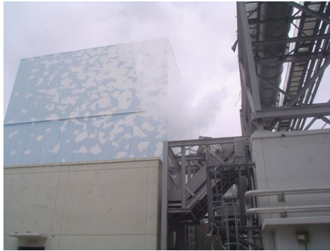
Figure 3 Steam coming out of a blow-out panel opening at the Fukushima Dai-ichi Unit 2 Reactor Building on March 15, 2011
